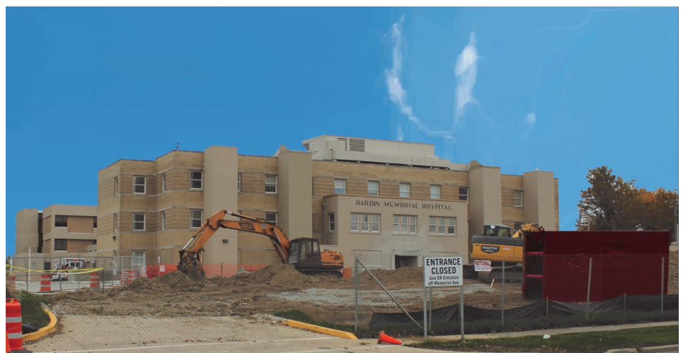
Hardin Memorial Hospital's expansion and renovation of its Emergency Department underway
