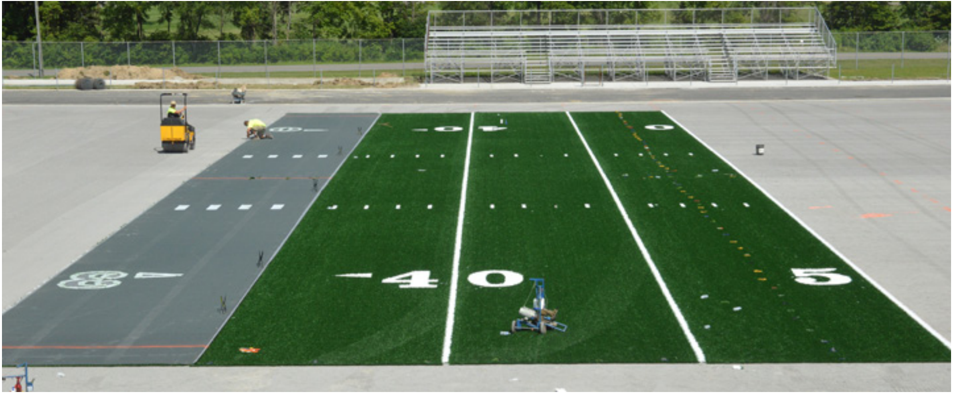
July - Artificial turf installed
